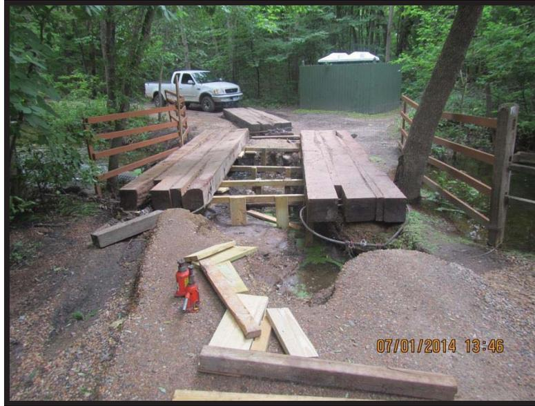
**FIGURE 10 KICIYAPI CULVERT CROSSING DURING EMERGENCY REPAIR**
