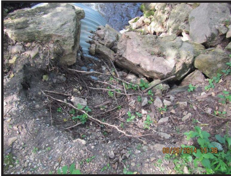
**FIGURE 18 EROSION AT SERVICE TRAIL CROSSING AFTER FLOOD**
