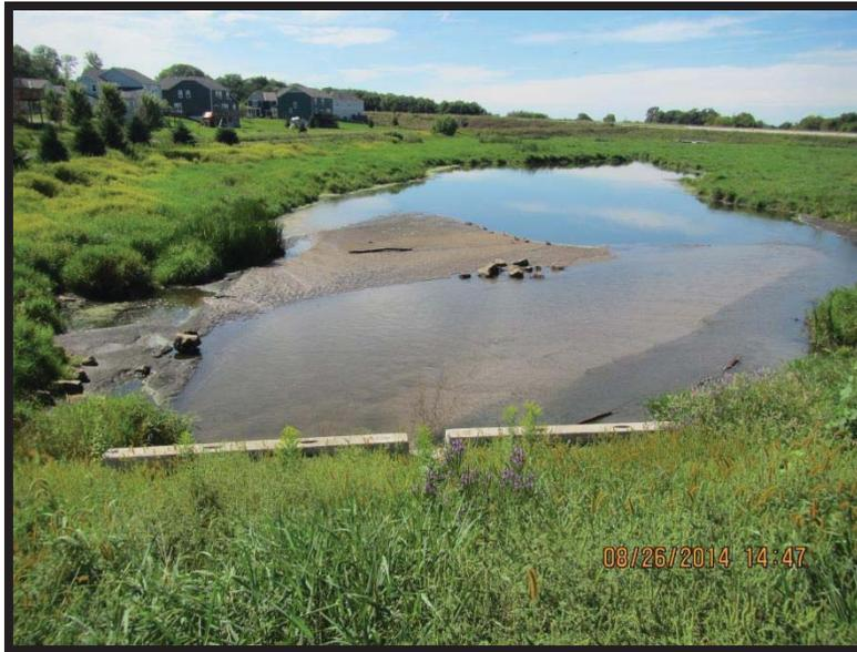
**FIGURE 16 SEDIMENT DELTA IN SEGMENT 5**
