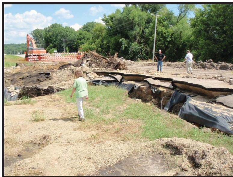
**FIGURE 15 COUNTY ROAD 16 AFTER FLOOD DAMAGE**
