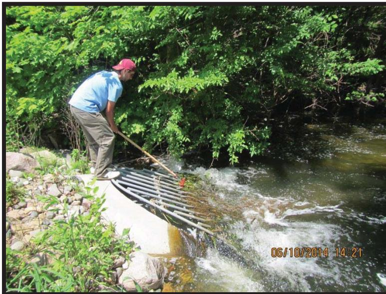
**FIGURE 19 REMOVING VEGETATION FROM CULVERT GRATE AT CR42**
