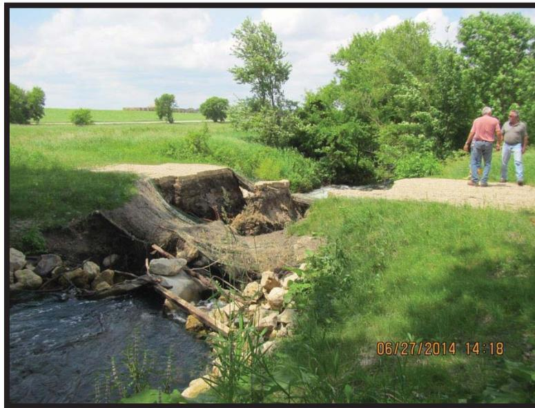
**FIGURE 14 GONYEA CULVERT AFTER FLOOD**
